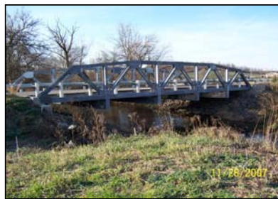
Bridge 173-0.12 over the Mad River
